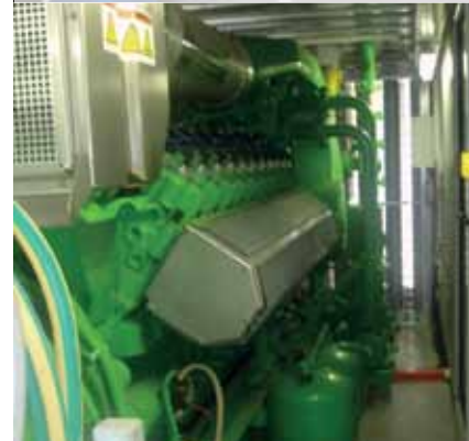
➤ Ecomax® interior, endothermic motor
