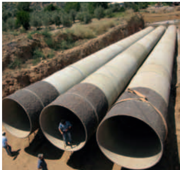
Joint and Wall Collar Sanded Circumferentially
