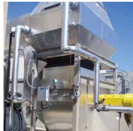
Secondary heat recovery system on an oxidizer.
