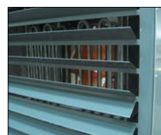
Detalle deflectores. View of deflectors.
