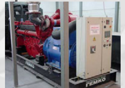
Emergency Stand by Generators 1500 KVA
