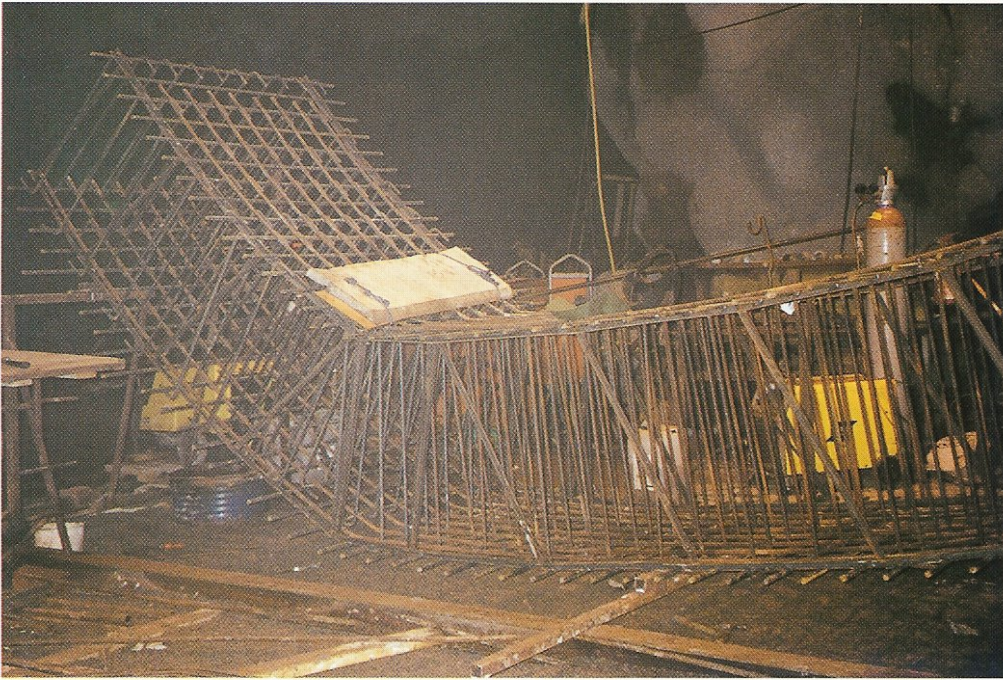
8 The final lining reinforcement cages being pre-fabricated before being erected in the next concrete lining pour
