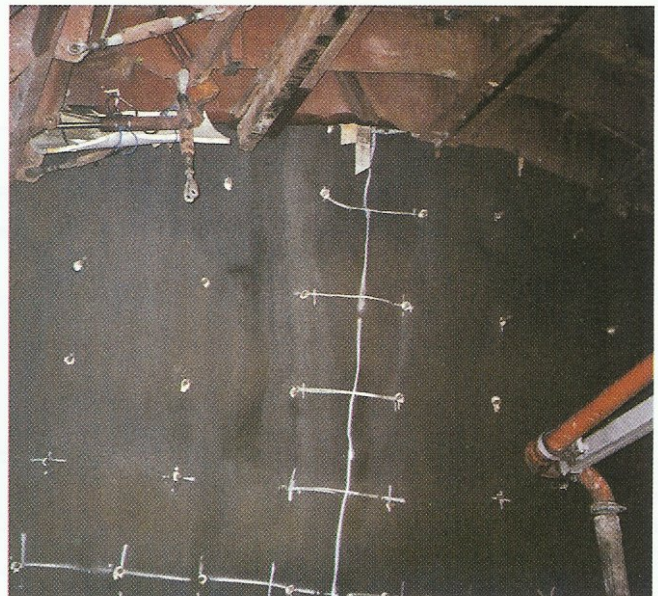
10 The shotcrete-covered face of the frozen zone with the charge holes drilled and the formwork of the previous concrete pour just 70 cm behind
