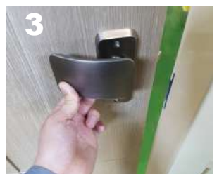
The door will be open at the same time as push the lever
