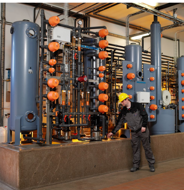
Boiler make-up water for high-pressure steam turbine.
