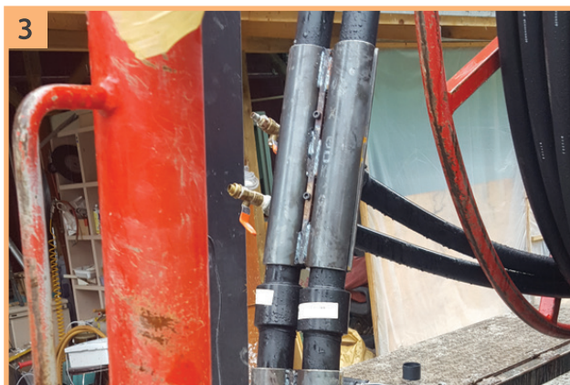
[ Installation of the weight band ]
