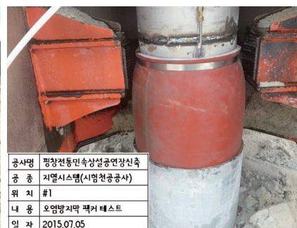
[ Contamination prevention (packer grouting) ]
