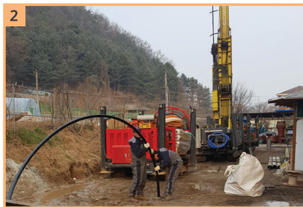
[ Installation of the ground heat exchanger ]
