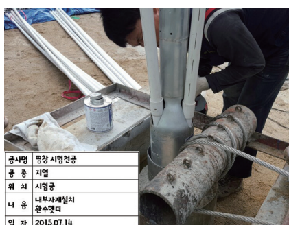
[ Recycled water pipe header installation ]
