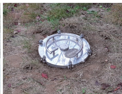
[ Close-type top protection hole installation ]
