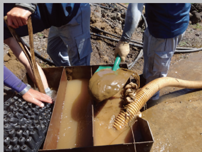
[ Looping route closure by sedimented materials ]
