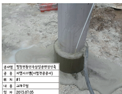
[ Contamination prevention grouting ]
