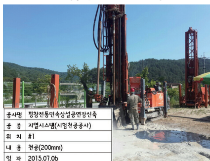
[ Geothermal borehole excavation ]
