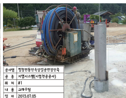
[ Lower fixing grouting ]
