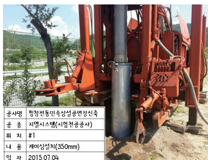
[ Installation of earthen block casing ]
