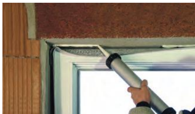
Installation example: ISO-TOP FLEX-ADHESIVE SP
