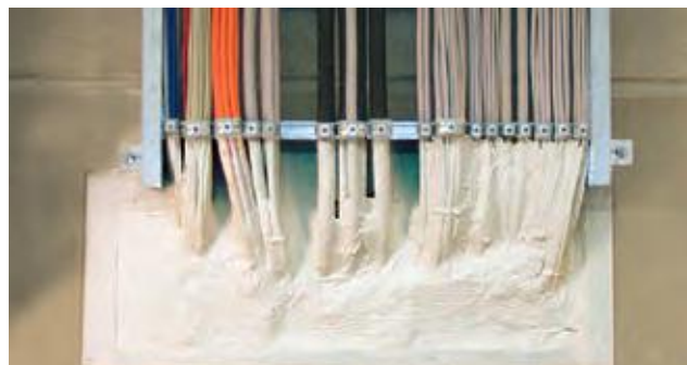
Installation example: ISO-FLAME BRICK S 90
