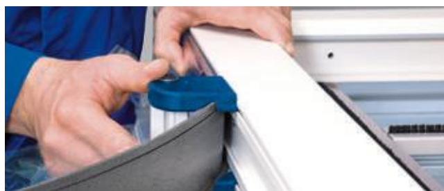
Installation example (CB): Fitting PVC windows
