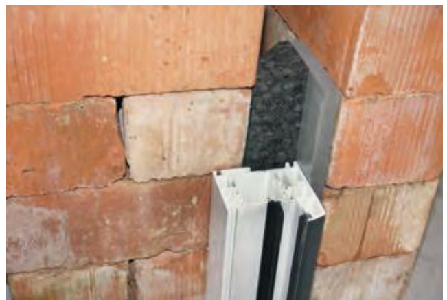
Installation example: ISO-BLOCO FILLER
