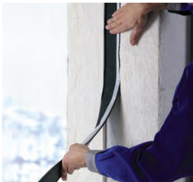
Installation example: ISO-BLOCO RENO
