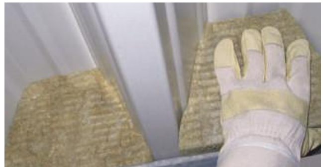
Installation example: ISO-PROFIL FILLER PIECES
