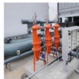
[Hyosung Heavy Industries Ara Waterway Logistics Center]
