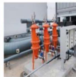
[Hyosung Heavy Industries Ara Waterway Logistics Center]
