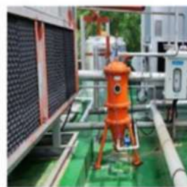
[Namyang Dairy's Gyeongju Plant]
