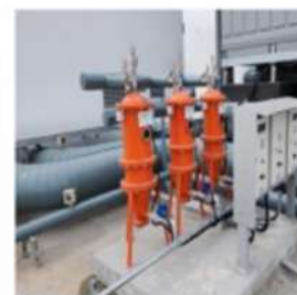
[Hyosung Heavy Industries Ara Waterway Logistics Center]
