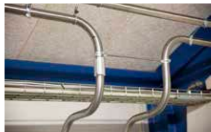
We provide you with a turnkey solution including installation work such as piping.
