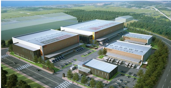
Seoul(Incheon) International Airport Duty Free Warehouse (Incheon, Korea) MIRINE® Indoor Ductless 106 units | 2014. 7.
