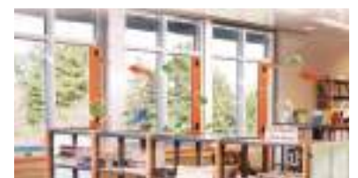
Window ERV installation
