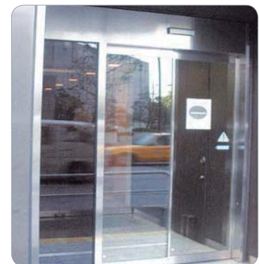
Entrance door in building 건물 출입문
