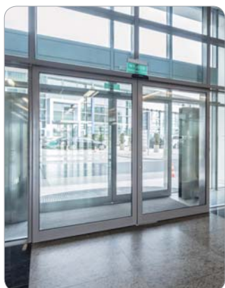
Entrance door in building 건물출입문
