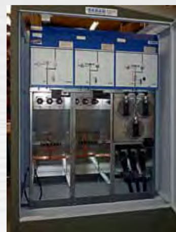
Tecnel MOZAMBIQUE - ORMAZABAL CGM 36kV utomhusstation
