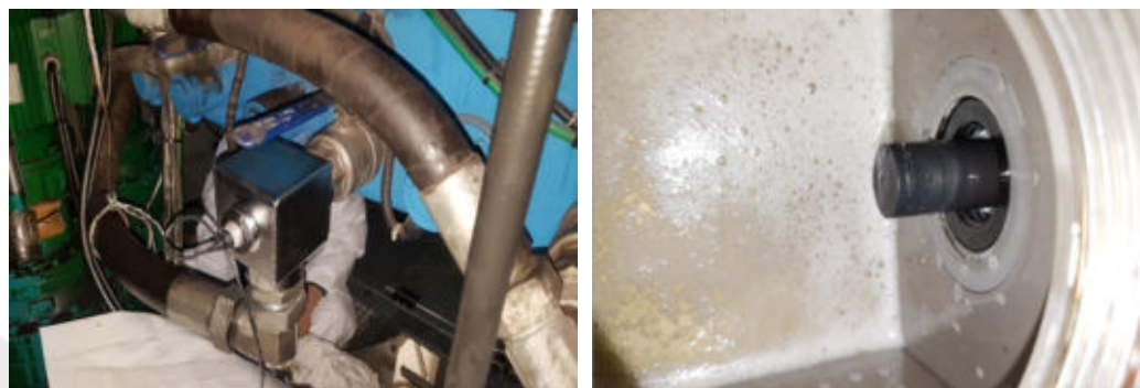
[Wind Turbine Gearbox]
