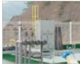
Elimination of VOC and bad odor
