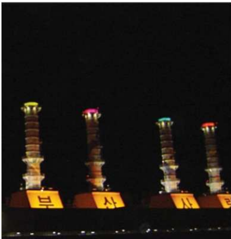
한국남부발전(주)부산복합화력발전본부 Korea Southern Power Combined Cycle Power Plant
