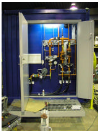
Fig.2. The reducing and supervising gas train in the wagon.
