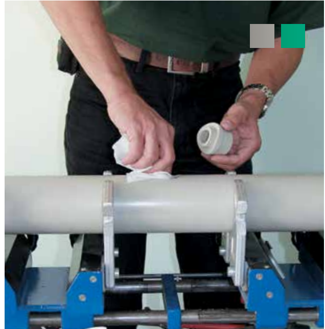
2. Clean. If you use the Stabi pipe, chamfer the edge of the drilled hole. Clean and degrease the weld-in saddle as well as the drilled hole.
