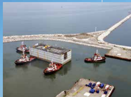
The final section of the flood barrier is towed into place.
