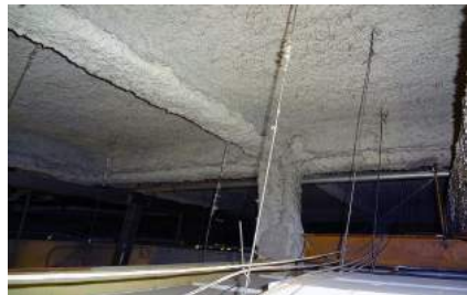
Plastering work of insulation (fireproof spray coat)
