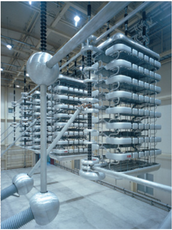
21st century ABB HVDC valves convert electricity from AC to DC, and vice versa Photo: ABB
